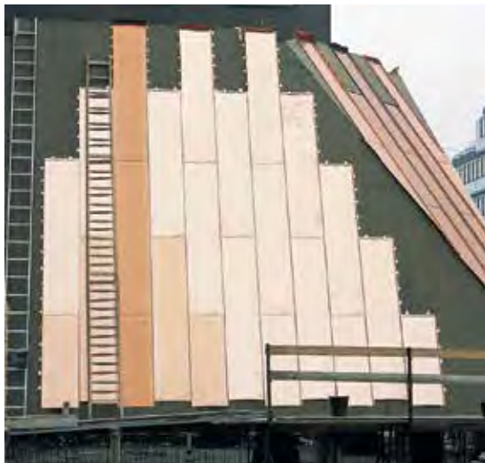
It is important for the substrate to be flat.
