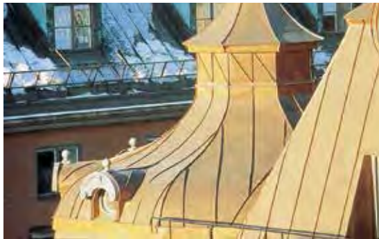
When designing details and connections to be attached to other materials, all the working is done manually. A stable substrate is required.
