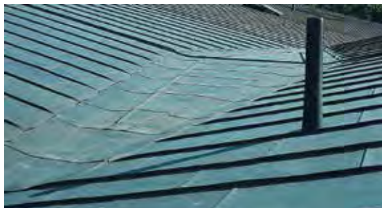
Is the valley tight? Are there any cracks in it, or any other damage?
