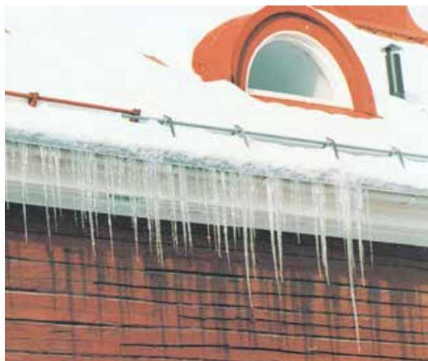
Icicles on the eaves indicate that heat is leaking out.
