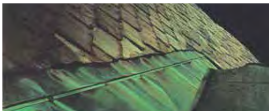
Sacrificial plate on a roof. To prevent erosion corrosion.
