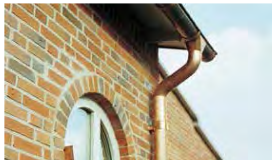
Is the downpipe union piece attached to the wall?
