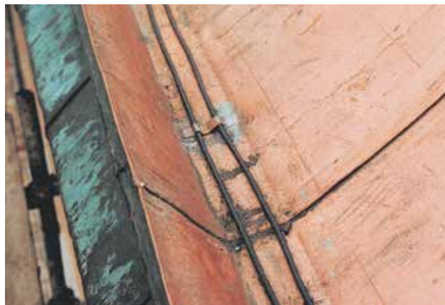
The formation of ice on the eaves can be prevented to some extent by using a heating cable, but it is important to design the roof initially in such a way as to prevent the formation of ice.
