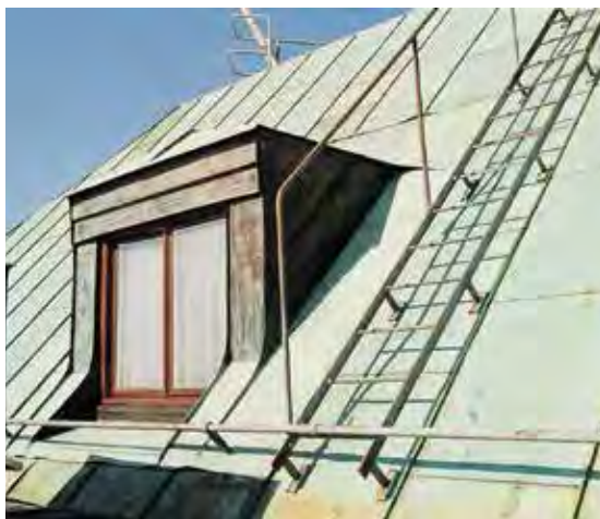
Checking the roof safety devices is a vital part of the maintenance inspection.
