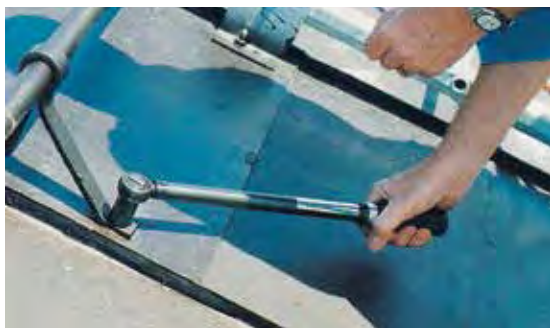
Roof safety device mountings in wooden bases must always be tightened. Lock joints, on the other hand, must not be tightened.
